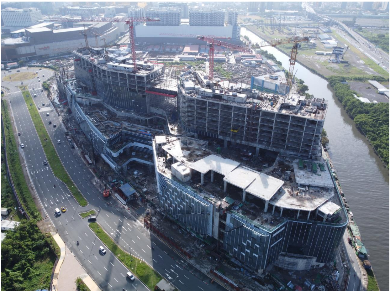
Figure 1 Construction progress at Westside City Project in August 2023
